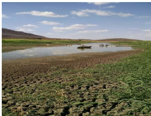
Figure 3 - Lucrécia Dam (RN), 2015.
