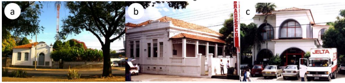
Figure 3 - a) Mrs. Elvina Ferraz Martins' residence; b) Manufacturer Álvaro Freire's residence; c) Governor Leônidas Melo's bungalow.
