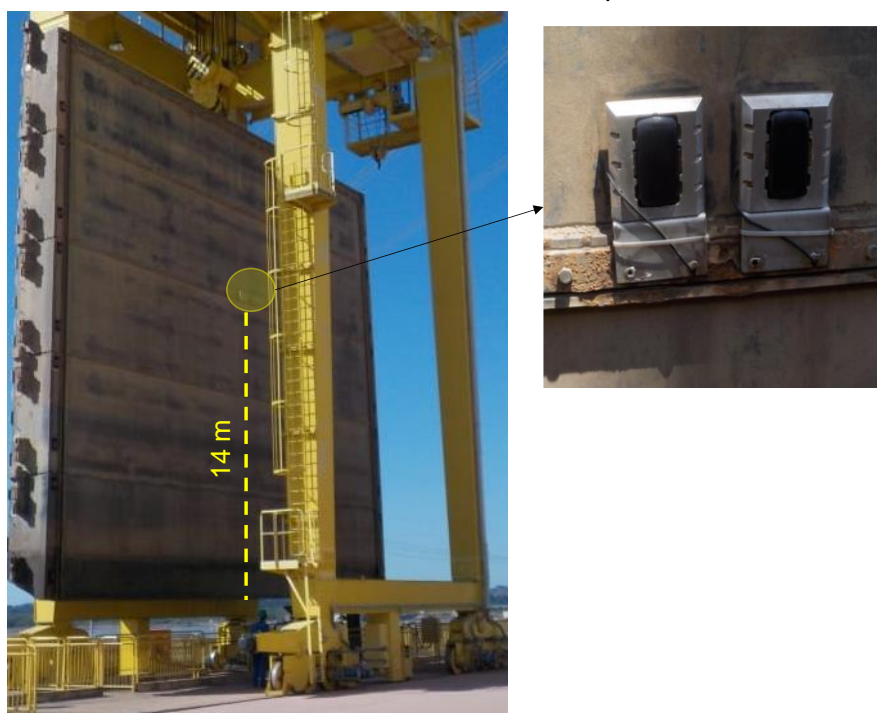
Figure 2 – Hydroacoustic system fixed to the gate at Jirau HPP (Patent no. BR 102015000457-5 A2 / www.venturoconsultoria.com.br ).
