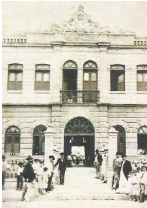
Figure 3 - Rui Barbosa Village - facade to the Senate Street
