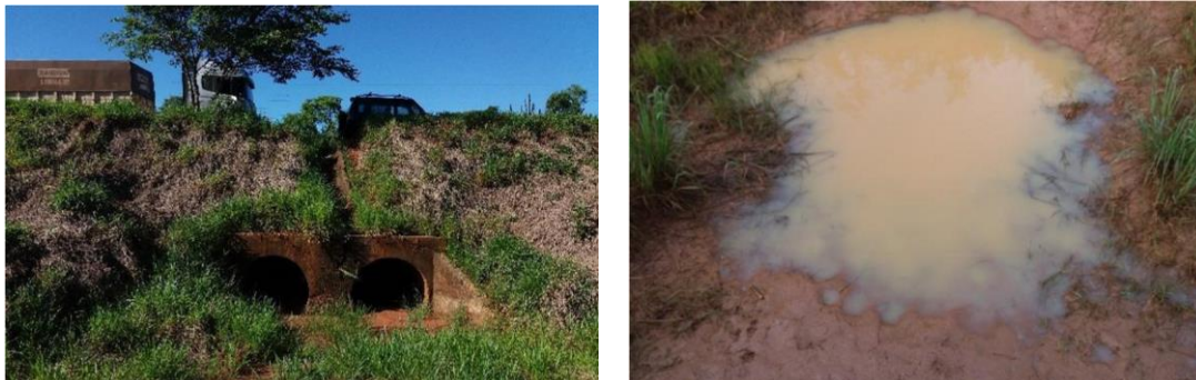
Fig. 5: Wild animals passages 1,45m in diameter under SP-613 highway inside MDSP, with formation of rainwater puddles that attract animals.
