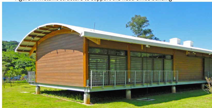
Figure 7: Metallic structure to support the head office building
