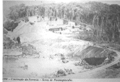
Figure 4 – Railway Construction Serra de Paranapiacaba /1860
