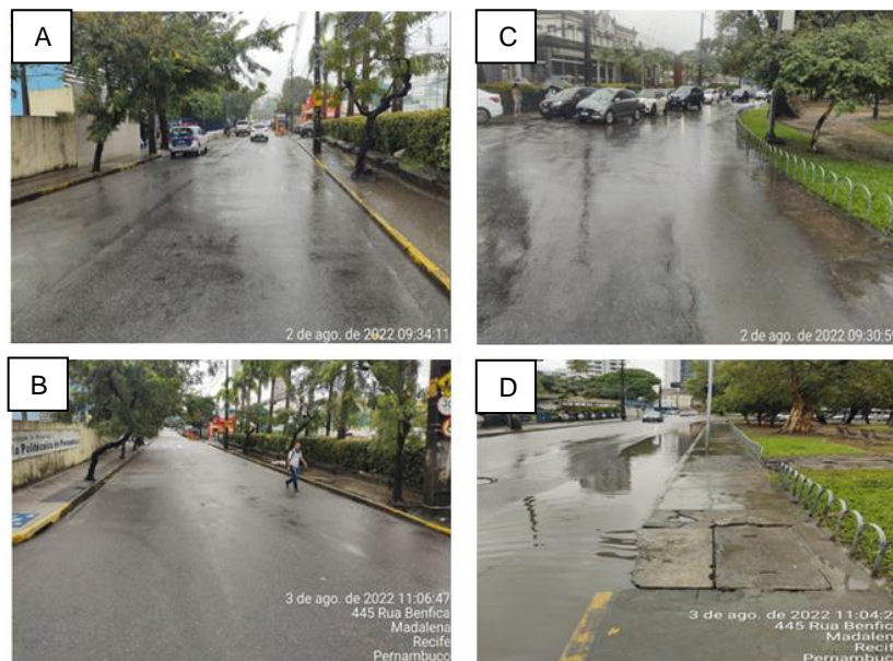
Figure 9 - Professor Benedito Monteiro Street, with normal flow of cars and pedestrians (A and B) and Benfica Street in front of the club, presenting vehicle retention due to water accumulation on the road (C and D), in the City of Recife.
