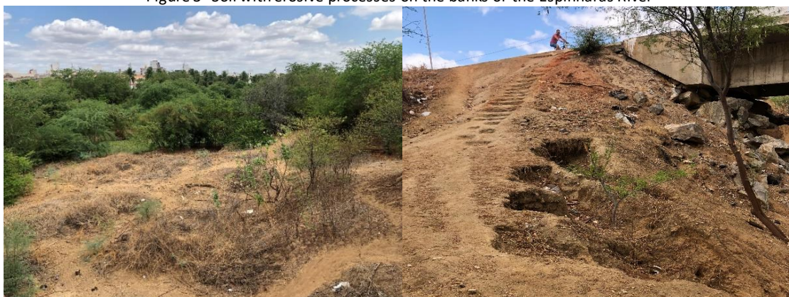
Figure 3- Soil with erosive processes on the banks of the Espinharas River
