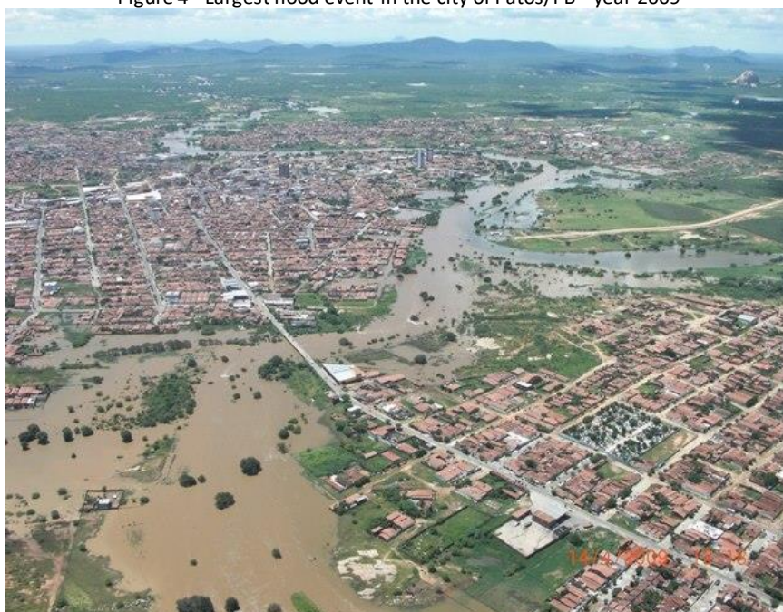
Figure 4 - Largest flood event in the city of Patos/PB - year 2009
