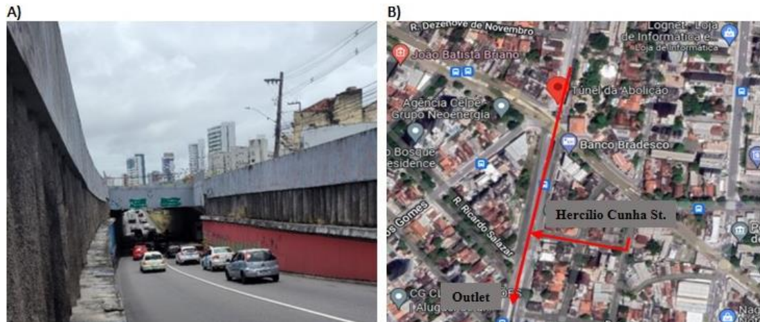
Figure 4 - A) Image of the Túnel da Abolição and B) its drainage network layout
