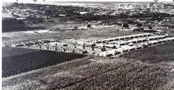
Figure 3 - Aerial photograph of the José Antonio Borelli Housing Complex in 1968.
