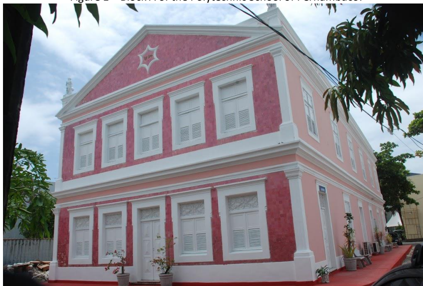
Figure 1 – Block A of the Polytechnic School of Pernambuco.
