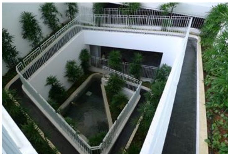
Figure 10 – Eco-cell system created by Ken Yeang as a way of reusing rainwater. From the images, you can see the path taken by the waters that are carried from the ramps and vegetated terraces by pipes to the eco-cell,
