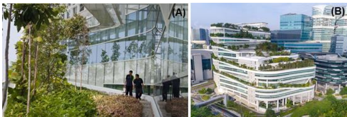
Figure 8 – Ecological ramp. (A) Operation of the ecological ramp with the space dedicated to vegetation and the maintenance walkway. (B) General panorama of the ecological ramp that runs along the building.
