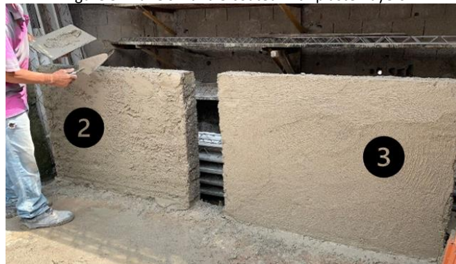
Figure 3 - Panels 2 and 3 coated with plaster layers
