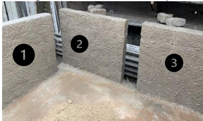
Figure 2 - Panels coated with a scratch coat layer.
