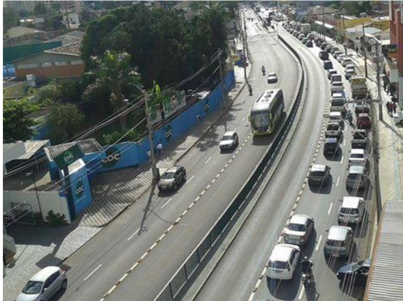
Figure 4: BRT system at Leopoldino de Oliveira Avenue
