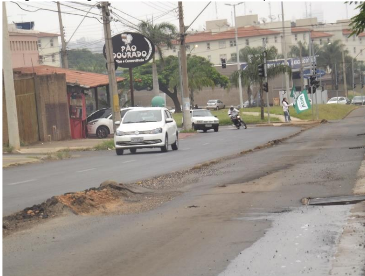
Figure 6: Paving of the BRT corridor on Avenida Leopoldino de Oliveira.
