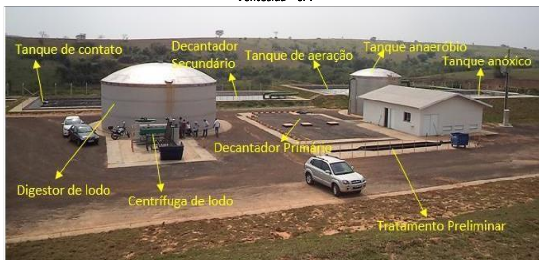
Figure 2 – Domestic sewage treatment equipment at the North domestic sewage treatment plant of Presidente Venceslau – SP .
