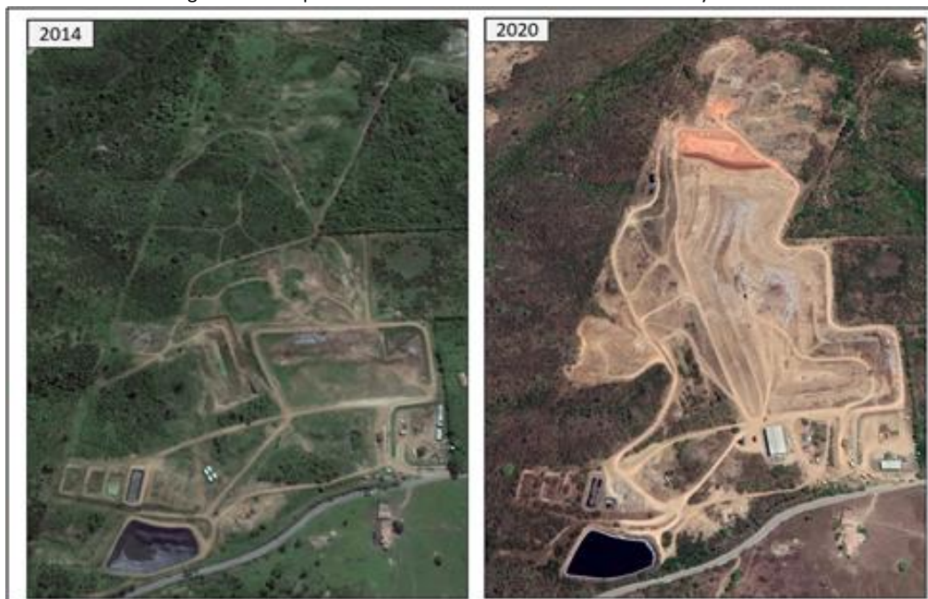
Figure 4 – Temporal evolution of the industrial waste sanitary landfill
