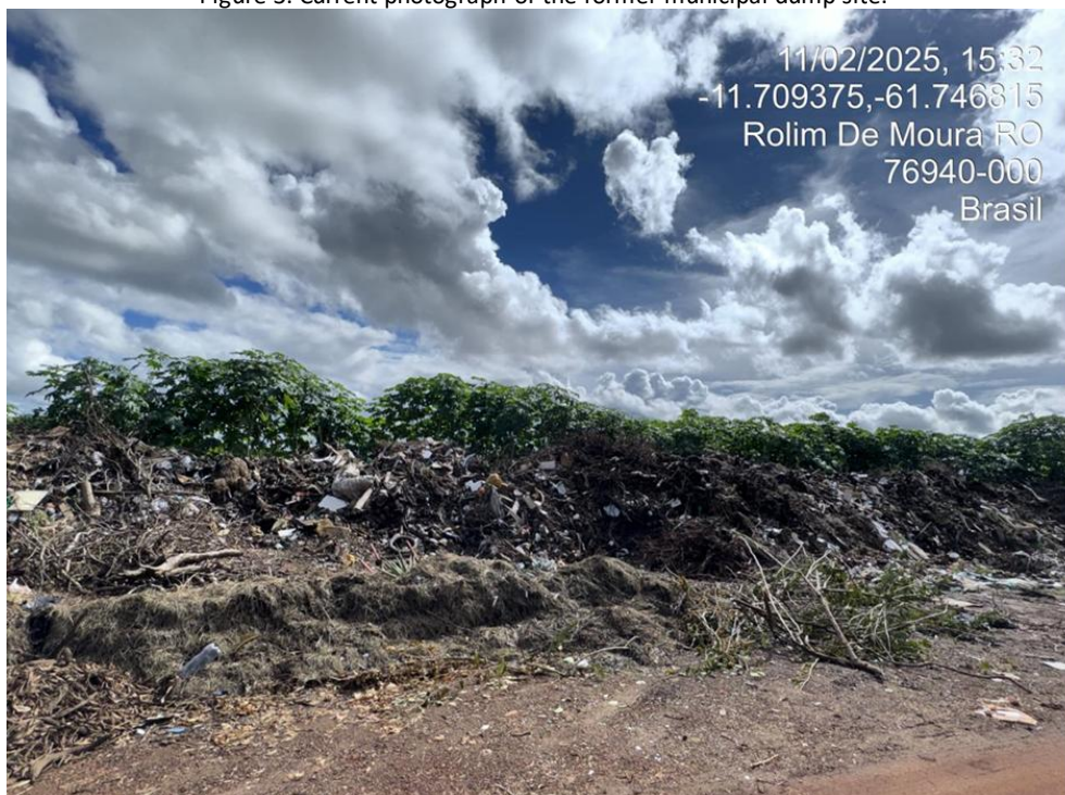
Figure 3. Current photograph of the former municipal dump site.
