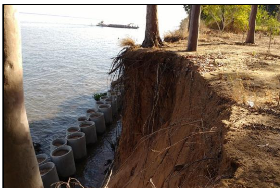
Figure 3 - Erosion process occurring on the banks of the Paraná River and containment barrier
