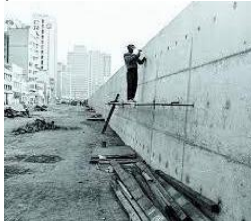
Figure 3 – Construction of the Mauá Wall in the 1970s
