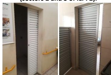
Figure 11: Inadequate access doors to toilets (sectors 2 and 3 of ILPI 2).
