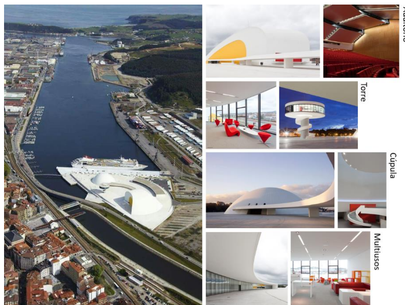
Figure 12. Aerial image and images of the buildings of the Oscar Niemeyer International Cultural Center
