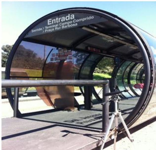
Figure 2: External view of a tube bus shelter and a B&K 2238 sound level meter mounted on a tripod
