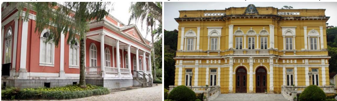
(b) View of the front façade of Palácio Rio negro , built in the eclectic style at the time of the Republic.
