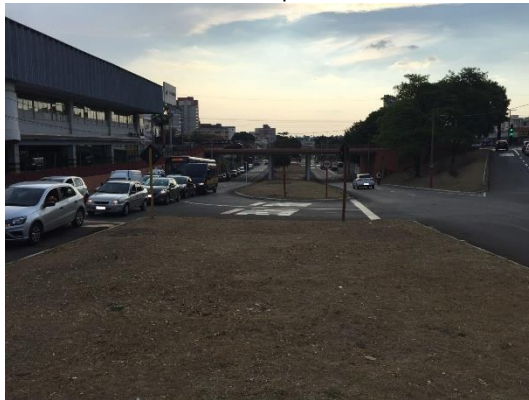
Point 10 - Trabalhador Sancarlense Avenue over the buried stream seen from upstream to downstream
