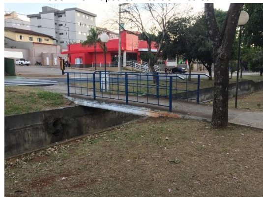
Point 12 - Pedestrian crossing over channelized stream seen from upstream to downstream
