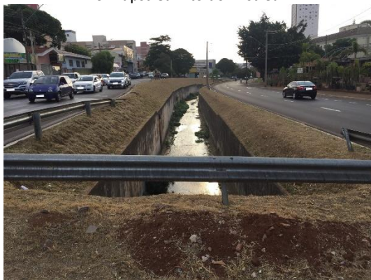
Point 11 - Transition between sections 2 and 3 seen from upstream to downstream
