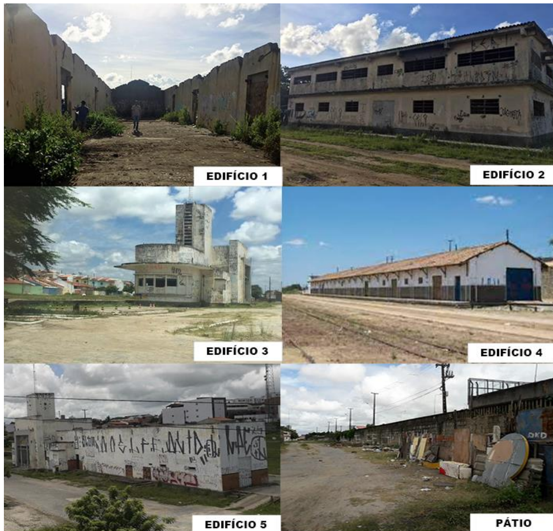
Figure 5 – Current situation of the buildings at the New Railway Station in Campina Grande.
