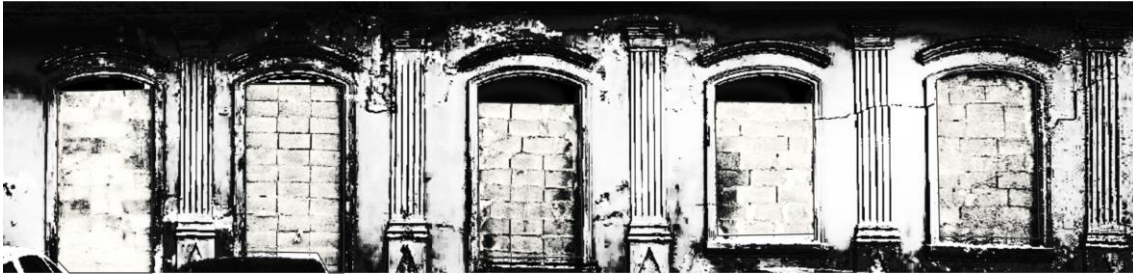
Figure 11 - The covered windows.
