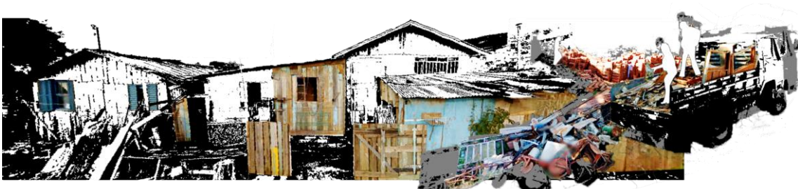
Figure 9 - The demolition of wooden architectures.
