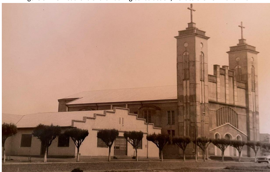
Figure 3 - New Catholic Church during construction, next to the new Parish Hall
