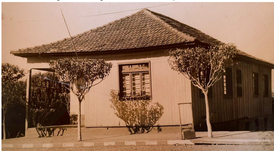
Figure 1 - Building that housed the first City Hall of Crissiumal
