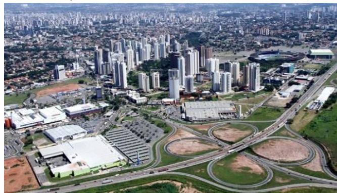
Figure 5: Jardim Goiás, in Goiânia, with emphasis on highways BR-153 and GO-020, and on large equipment and urban dynamics, such as verticalization and densification
