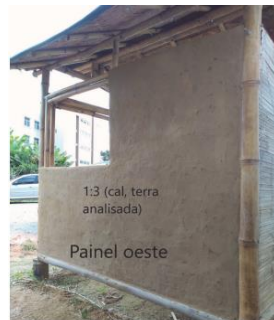
Figure 9 – Plaster application
