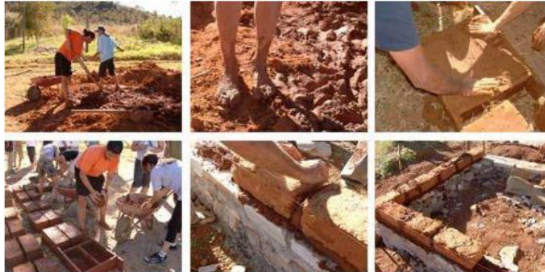
Figure 4—production of estrutural adobe blocks
