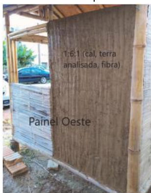
Figure 7 – Scratch coat application with lime
