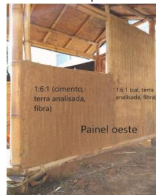
Figure 8 - Scratch coat application with cement
