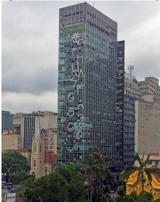
Figure 7 – Deterioration of the Wilton Paes de Almeida building
