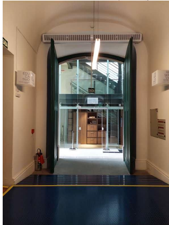
Figure 10: View to the annex with another material composition (glass and metal structure)
