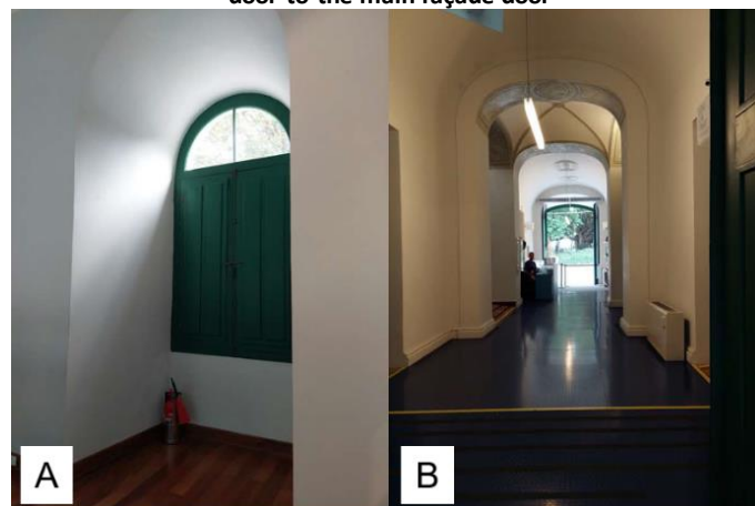
Figure 5: Entry of daylight into the building. (A) Glass in the upper part of the window (B) View from the back door to the main façade door
