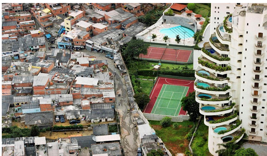
Figure 1 - Penthouse Building and Paraisópolis slum, São Paulo (SP)
