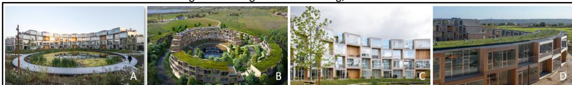
Figure 1 – Sneglehusene Housing, Denmark.
