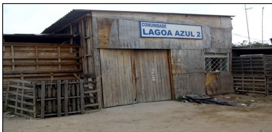
Figure 3: View of the Community Center of ``Lagoa Azul`` Community 2
