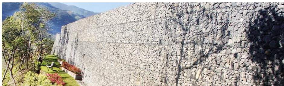
Figure 1- Containment structure made with basket gabion
