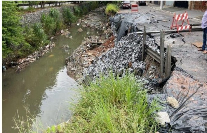
Figure 7- General view of the site and temporary containment.
