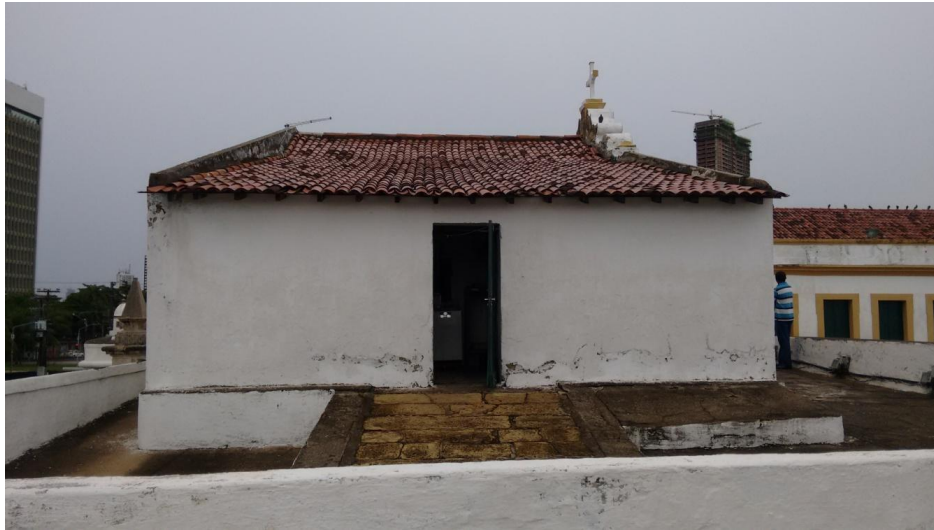
Figure 7: Current situation of the woodwork and roofing of the Brum Chapel
