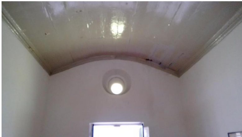
Figure 6: The ceiling seen from the altar. Note its deformation, giving the impression of a barrel vault rather than the bowl shape observed in the opposite direction.
