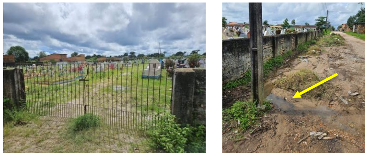
Figure 7. Surface water runoff at the Campo da Saudade cemetery, Bragança, Pará.
