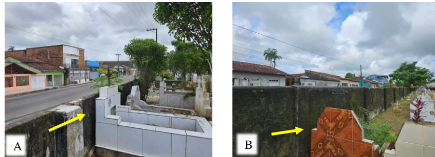
Figure 8. Setback of less than five meters in relation to the cemetery perimeter: A – Santa Rosa de Lima and B – Campo da Saudade, Bragança – Pará.
