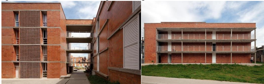
Figure 8: Circulation between buildings – footbridges.
