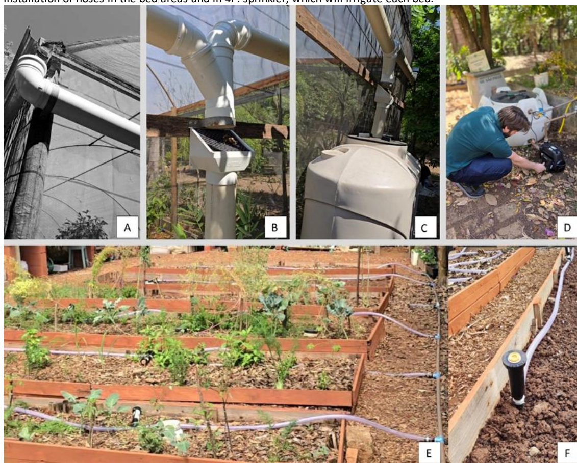
Figure 4. Images demonstrate the execution of the rainwater harvesting project at Horta das Flores for irrigating PANC (non-conventional food plants) beds. In 4A: gutter installation; 4B: junction of pipes from the side gutters of the greenhouse; 4C: collection reservoir; 4D: reservoir that will distribute water to the 10 beds and the pump; 4E: installation of hoses in the bed areas and in 4F: sprinkler, which will irrigate each bed.
