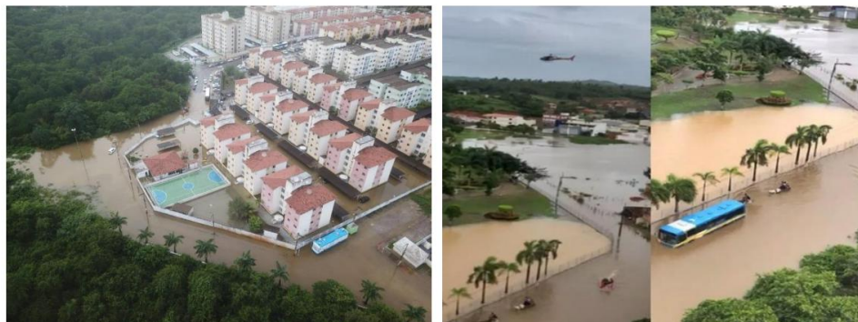
Figure 5 - Floods in Jabotiana neighborhood.
