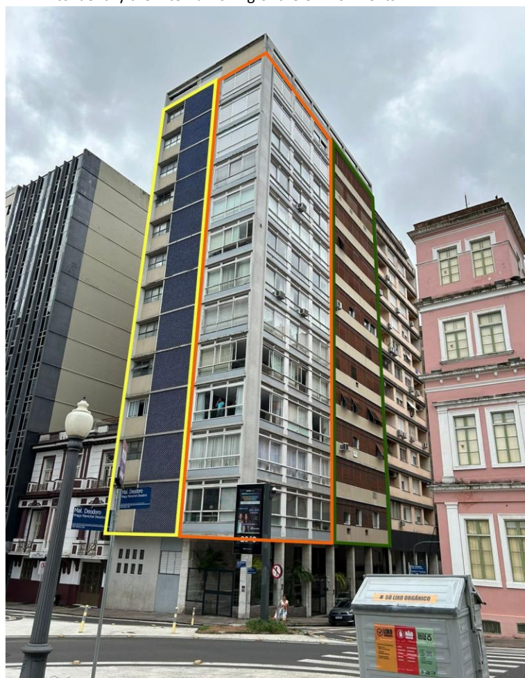
Figure 08 – Mapping of the different façade treatments present in the Faial building that make it possible to identify the internal zoning of the environments.
