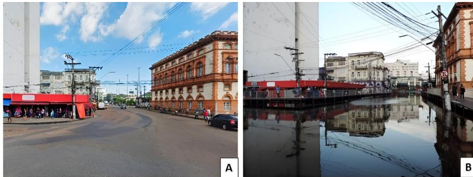
Figure 8 – Floriano Peixoto Avenue, built over the bed of the Igarapé dos Remédios.
